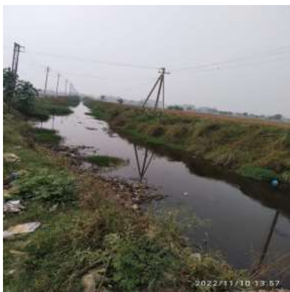
Figure 88 Bhoorgarhi – Kalugarhi confluence drain
