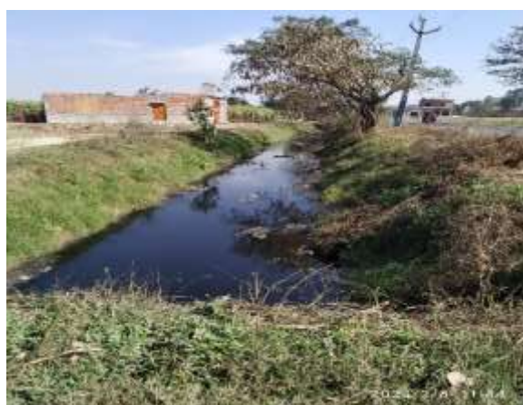
Figure 60 Mansoorpur drain near Husenpur Bopara village
