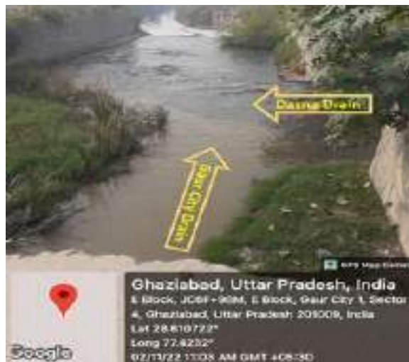
Figure 95 Dasna and Gaur city drain
